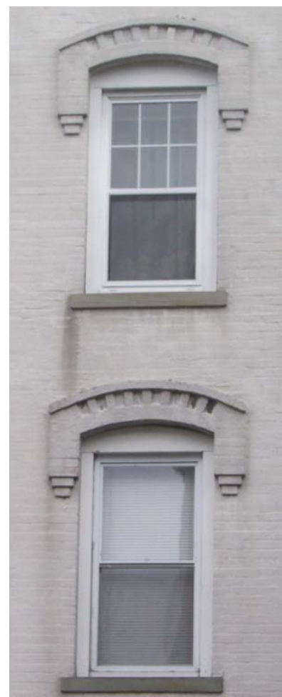
Not Recommended: Using sash with inappropriate division of panes. The upper-sash with new 6/1 sash does not match with the lower 1/1 sash.
