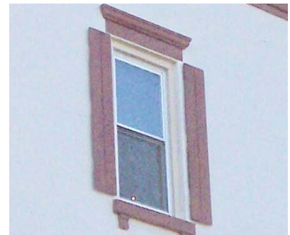
Not Recommended: Using shutters where there is no evidence for their historic use and that are too narrow and so clearly cannot function.
